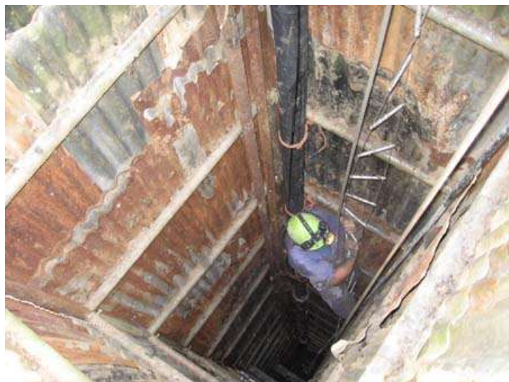
Descending shored shaft during excavation of a Limestone mine in Sussex.
