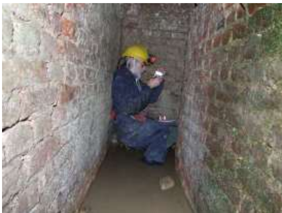
Surveying Tudor Drain at Roydon Hall, East Peckham
